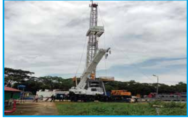
Kailashtilla well no. 1 workover project.
