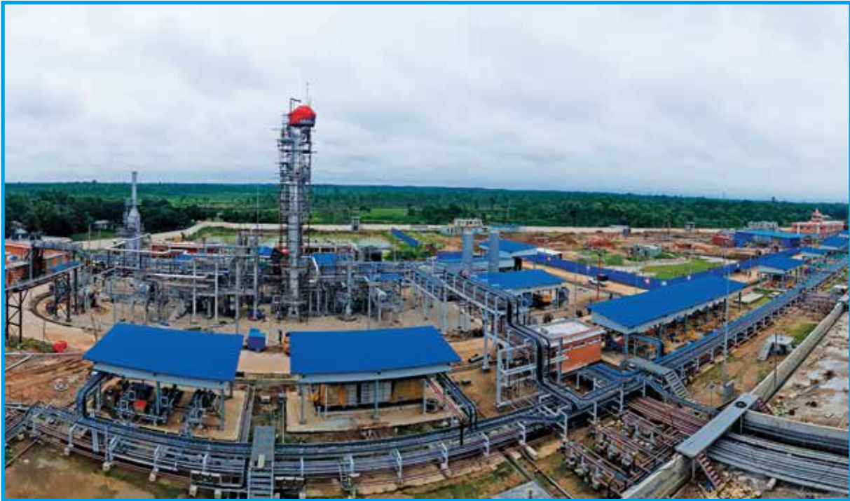
Process area and pump shelter of 4000 bpd
