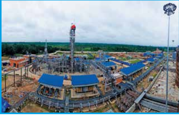
Process and pump shelter of 4000 bpd CFP Project.
